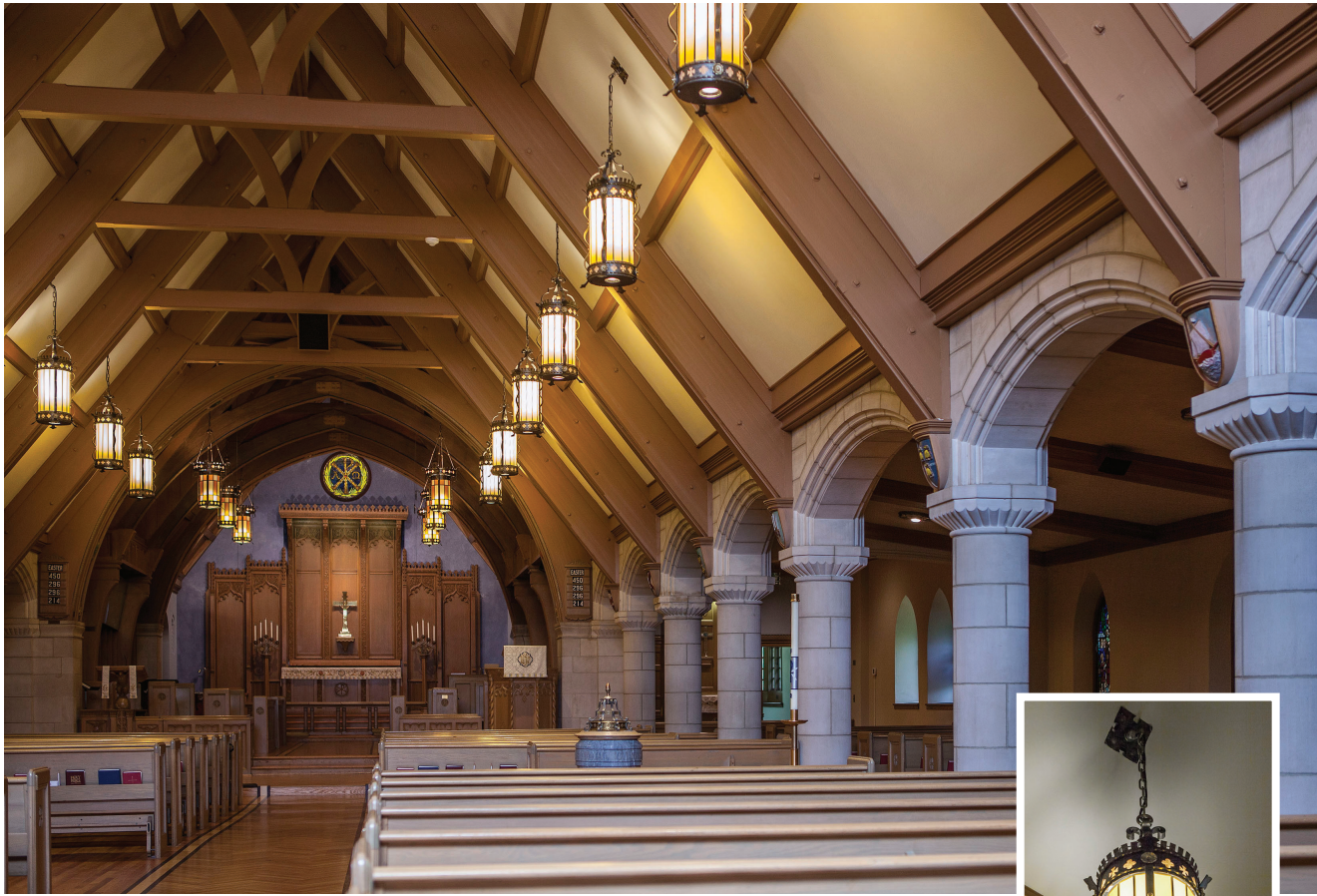
At Christ Church in Short Hills, NJ, pendant lanterns are fitted with LED uplights and downlights.
